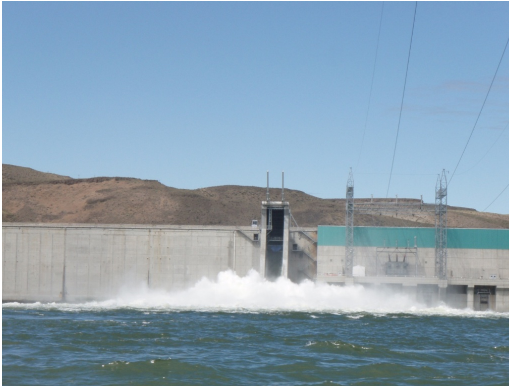
Figure 5 Wanapum Fish Bypass facility, mid-Columbia River, WA.
