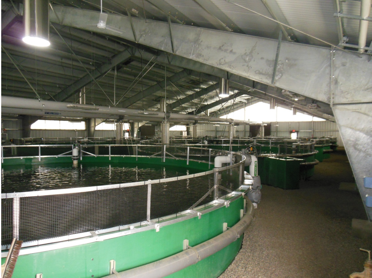
Figure 9 Carlton Acclimation Facility rears Methow summer Chinook using eight 30-foot diameter round tanks.
