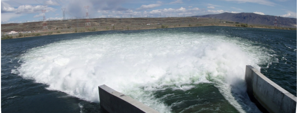
Figure 2 Photograph of Wanapum Dam Fish Bypass facility, looking downstream, mid-Columbia River, WA.
