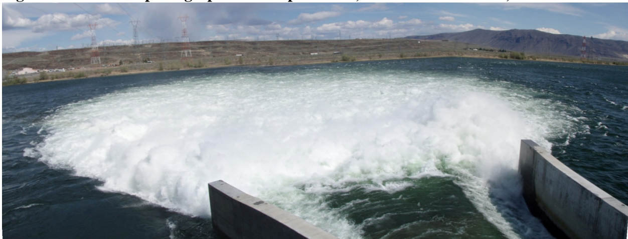
Figure 3 Photograph of Wanapum Dam Fish Bypass facility, looking downstream, mid-Columbia River, WA.
