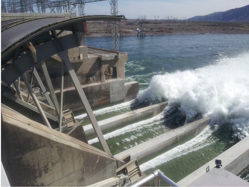
Figure 6 Photograph of the Priest Rapids Fish Bypass facility, mid-Columbia River, WA.
