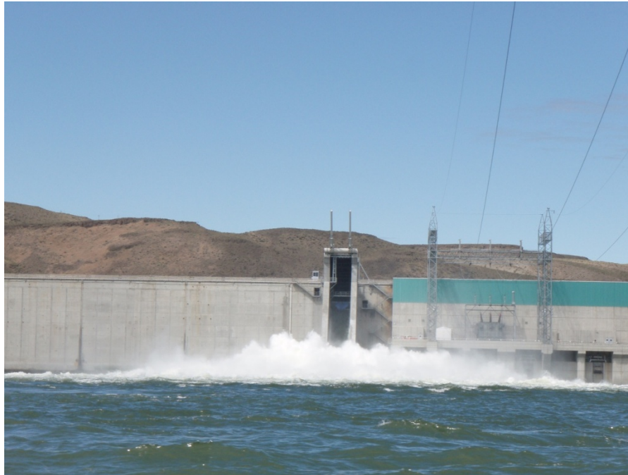
Figure 5 Photograph of Wanapum Fish Bypass facility, mid-Columbia River, WA.
