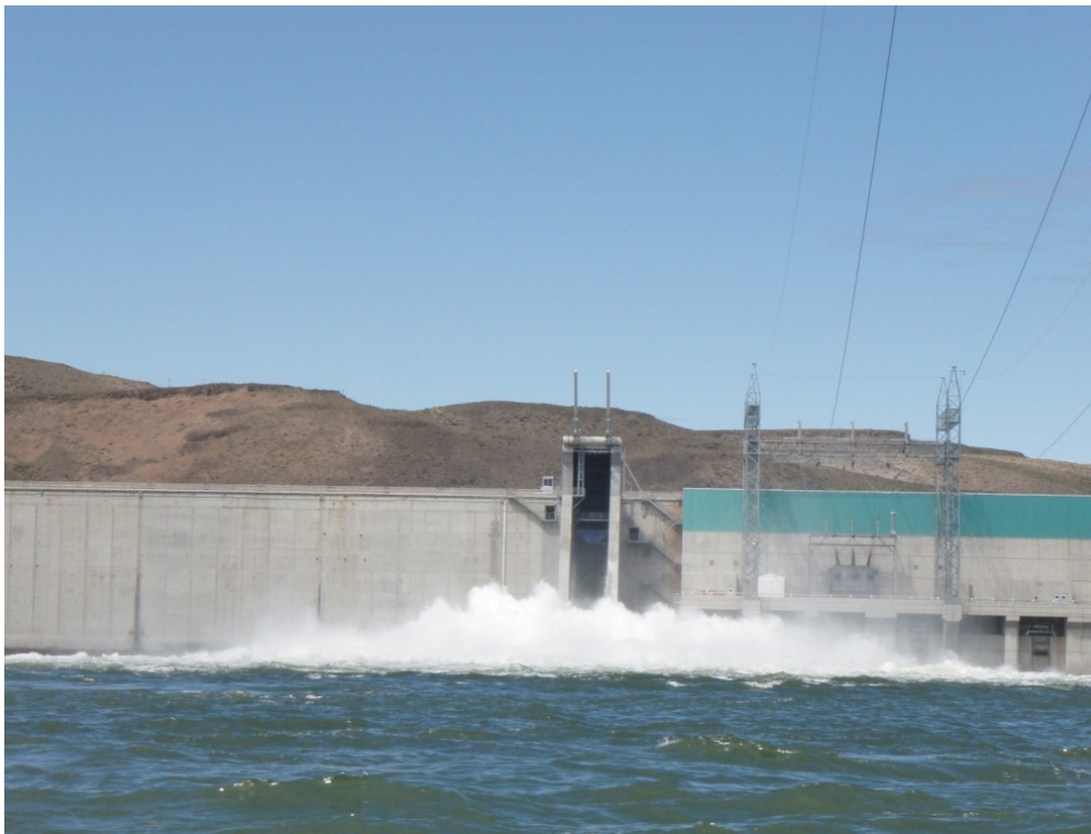
Figure 5 Wanapum Fish Bypass facility, mid-Columbia River, WA.
