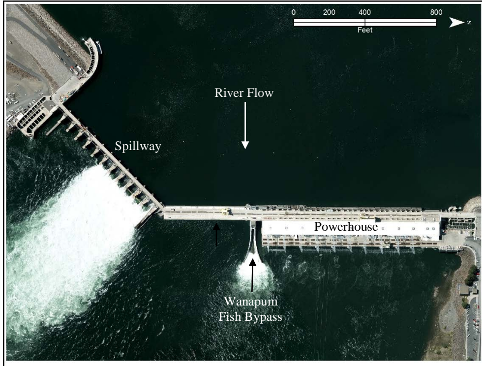
Figure 3 Aerial photograph of Wanapum Dam, Priest Rapids Hydroelectric Project, mid-Columbia River, WA.
