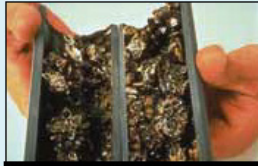
Zebra mussels in a cut-away pipe
