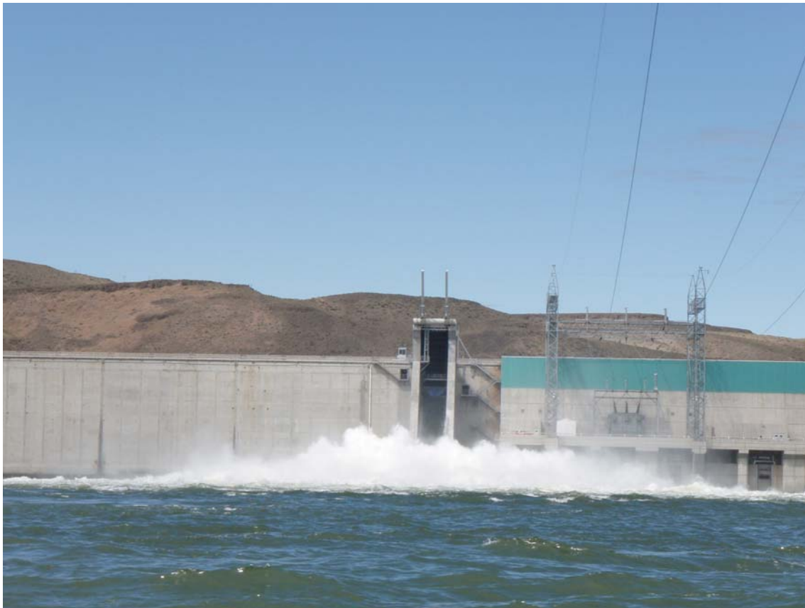
Figure 7 Photograph of Wanapum Fish Bypass facility, mid-Columbia River, WA.
