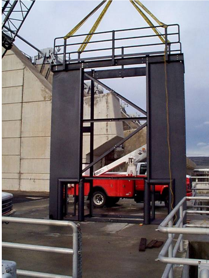
Figure 4 In-ladder box during assembly and installation at Wanapum Dam.
