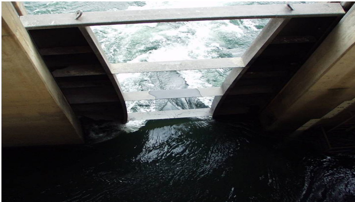
Figure 1 LSE-4 at Priest Rapids Dam, Columbia River mile 397.1, Washington, USA.
