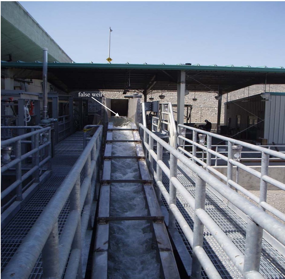
Figure 2 Steeppass Denil section of the off-ladder adult fish trap located at Priest Rapids Dam, Columbia River mile 397.1, Washington, USA.
