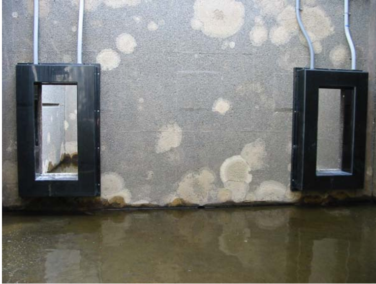
Figure 2 PIT-tag antennas mounted to the upstream face of Weir 3 in the Priest Rapids Dam east-bank adult fishway.
