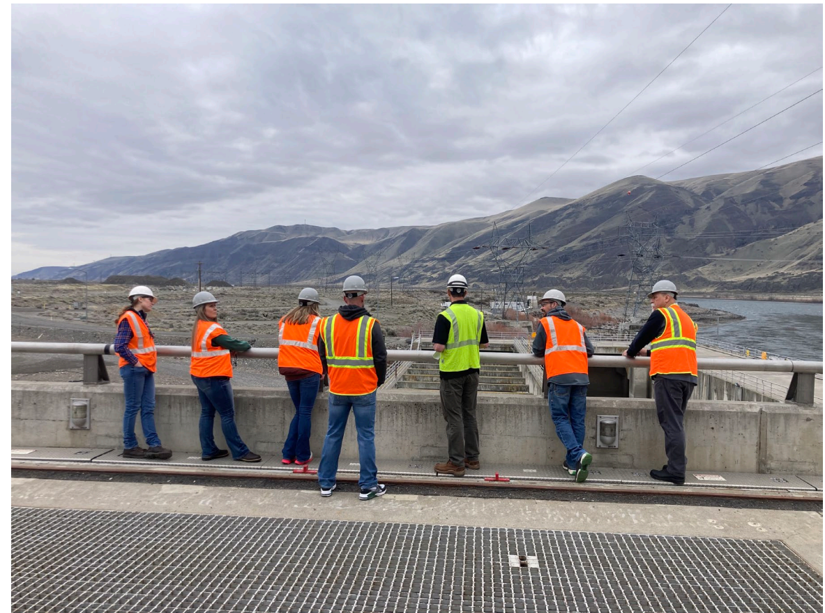
Photo taken at Priest Rapids Dam during the Power Production Tour.
